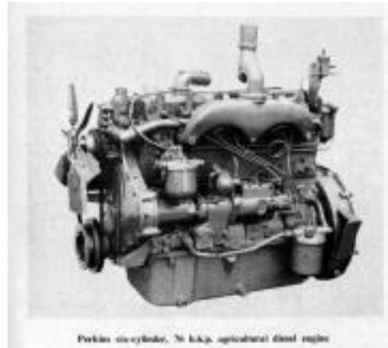
1959. Six-cylinder 76 b.h.p. agricultural diesel engine
